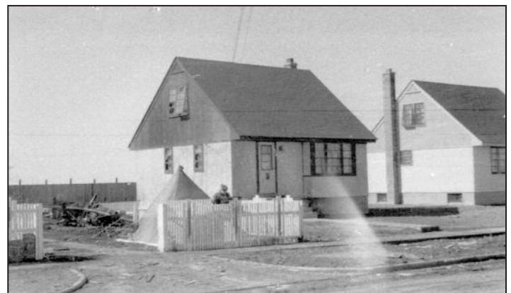
Wreckage in the back yard at 1330 3 rd Avenue. This house also sustained fire damage. Note the investigator's tent erected on the property.
