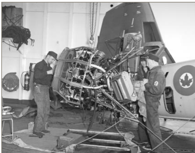
Arctic Engine Change of HUP Aircraft Onboard Labrador. Photo Source: DND Via Lt (P) J.A.MacNeil Collection
